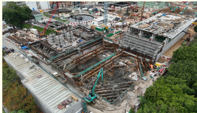
基本處理設施的挖掘及側向支撐安裝工程 Excavation and Lateral Support Works for Preliminary Treatment Facilities
