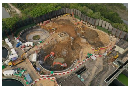
拆除現有最後沉澱池 Demolition of the existing final sedimentation tanks
