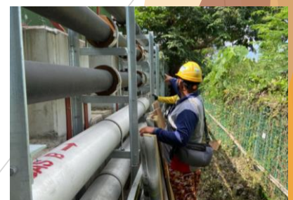
臨時管道改道工程 Temporary utilities diversion works
