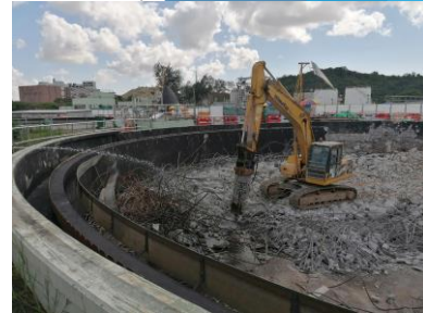
Demolition of primary sedimentation tank nos. 7 & 8 拆除7號及8號初級沉澱池
