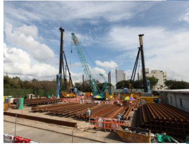
Piling works for Inlet Works 入水廠房打樁工程
